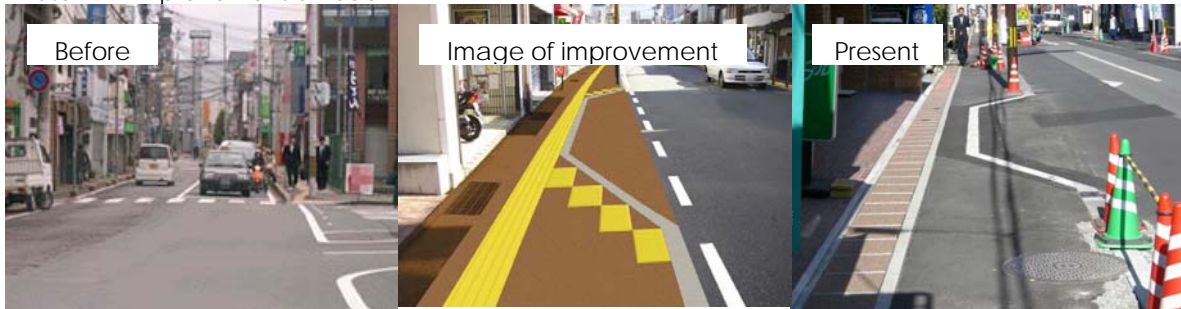
Photo 11 Improvement of road
