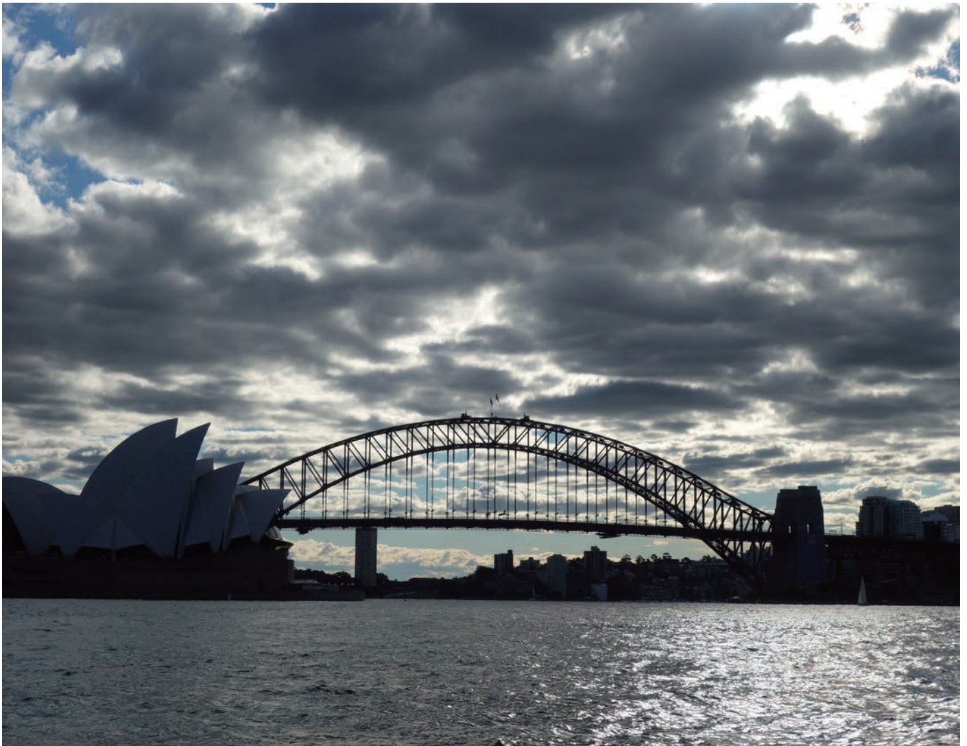
Sydney Harbour Bridge
